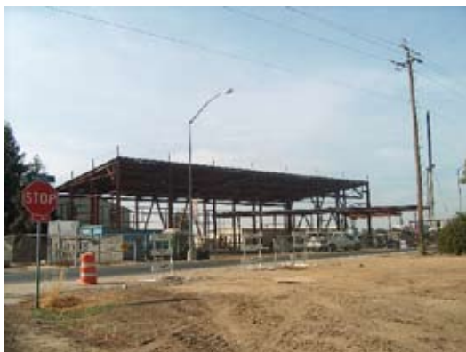
Right: Test and certification building floor prior to concrete pour, July 2006.
